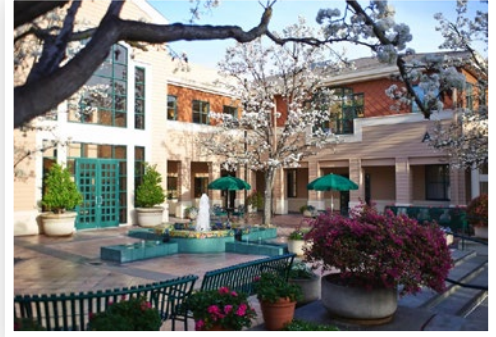
Front entrance to The Terraces
